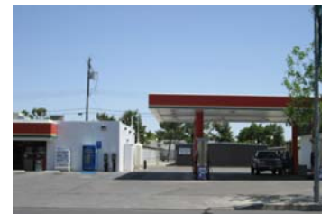
Traditional gas station in Zone 1
