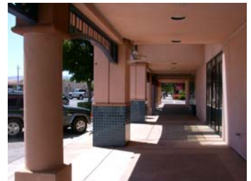
Arcade at City Hall, Zone 2.
