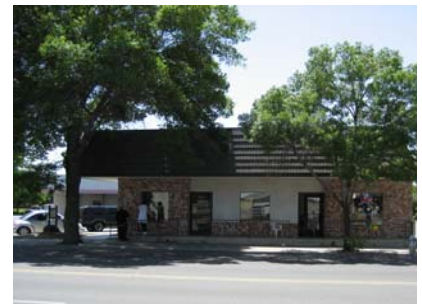
Store at curb line in Zone 4
