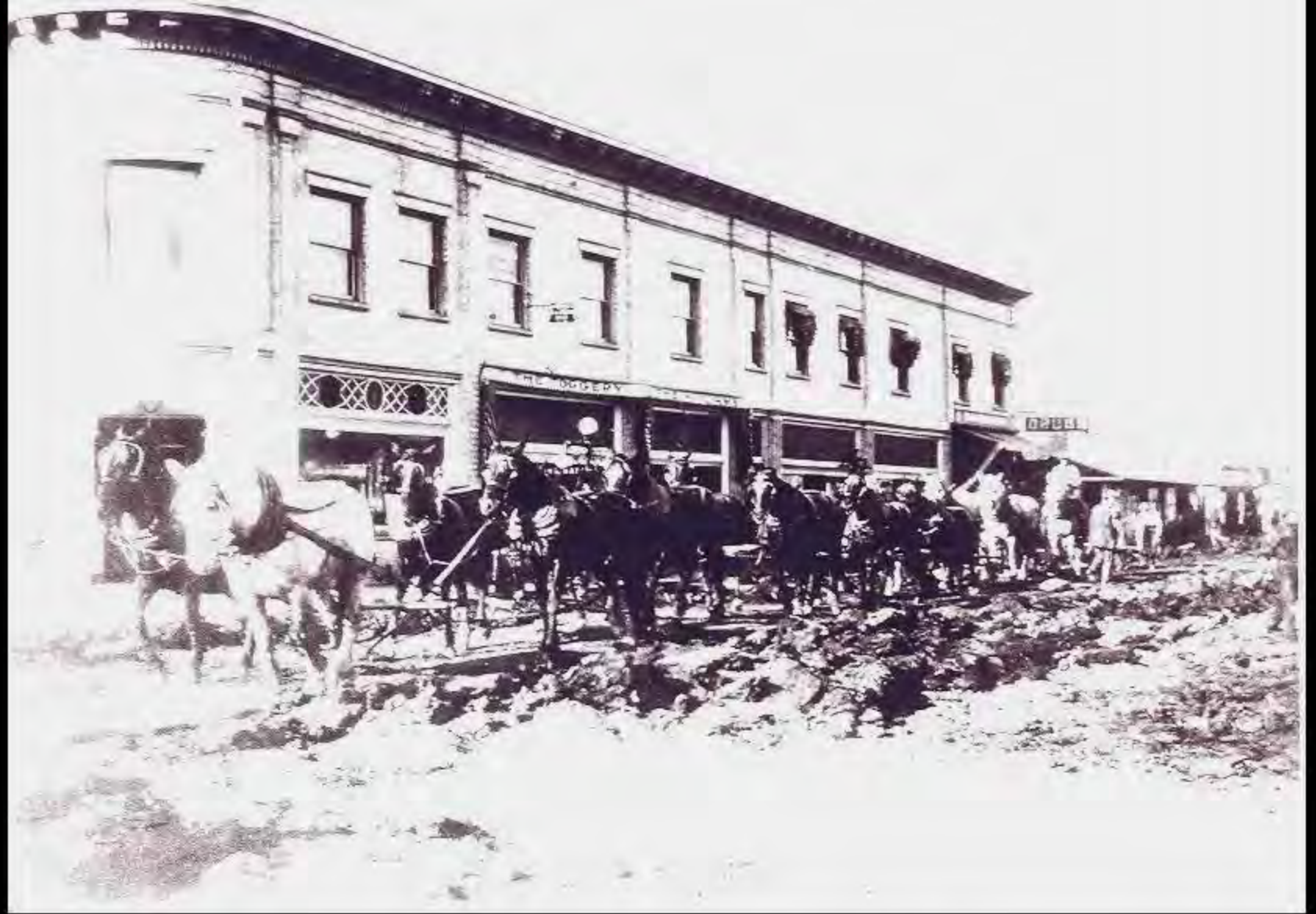
Street paving project 1917
